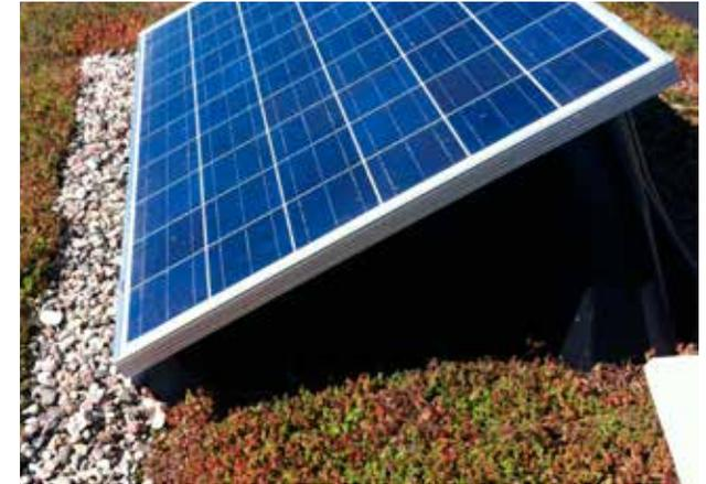
Solar cells can be incorporated nicely with establishment of a green roof.
