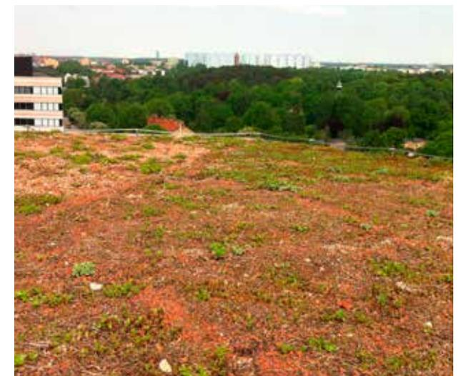
The K1 auditorium in Stockholm has a sedum roof. The main reason for choosing a green roof was to even out the stormwater load during heavy rain. (Photo: Eva Sikander)
