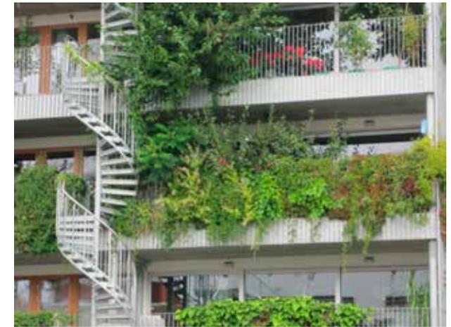
"Urban villas", Malmö. The balconies are reinforced for cultivation beds. There is 30 cm of soil under the floor boards. Any number of boards can be removed in order to access the soil for gardening. (Photo: Varis Bokalders)
